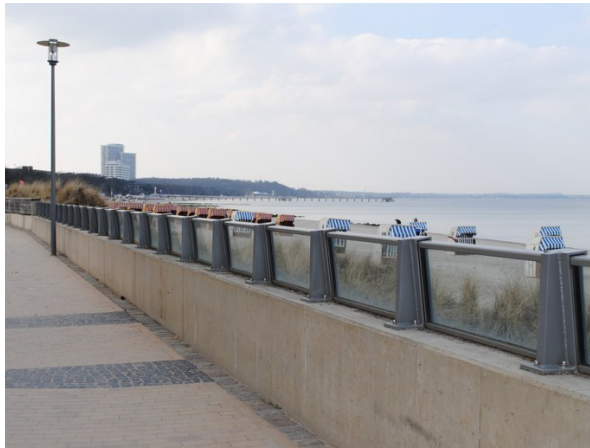
Figure 5.5 Timmendorfer Strand beach and design of the coastal flood defence measure (the glazed retention walls increase the attractiveness of the area for visitors and local citizens)
